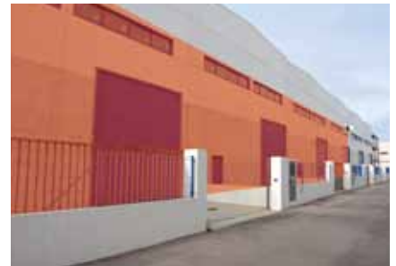
Wall protection (outdoor) at Warehouse
